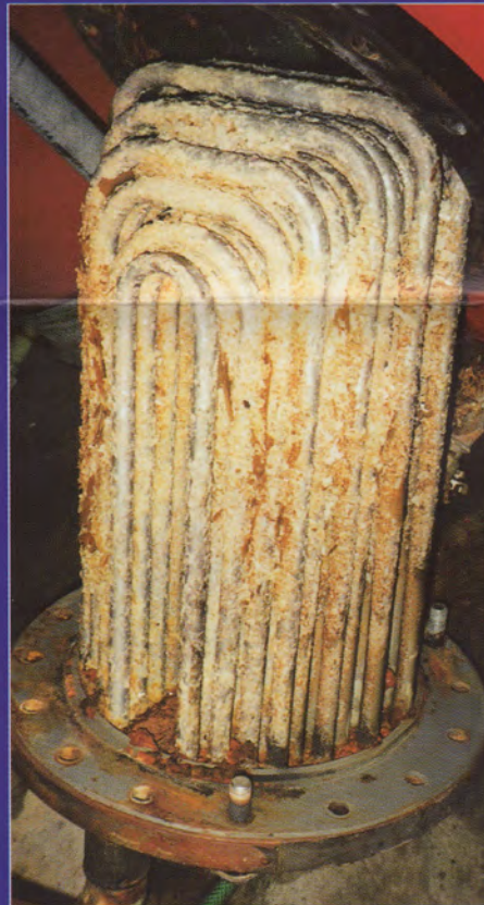
Heizelement Grossboiler
